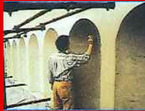
Coating with ancient render, protective treatment : INTONACHINO STORICO – IMPERM. WP55 – TECNOSOLID 82
