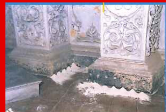
Coating with ancient render, protective treatment : INTONACHINO STORICO – IMPERM. WP55 – TECNOSOLID 82
