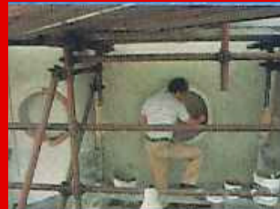
Coating with ancient render, protective treatment : INTONACHINO STORICO – IMPERM. WP55 – TECNOSOLID 82
